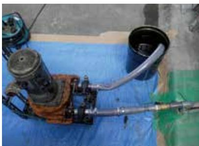
⑤止水充填材の充填
